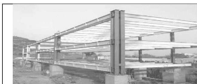
Fig.2 Erected Frame after 1st Lift
